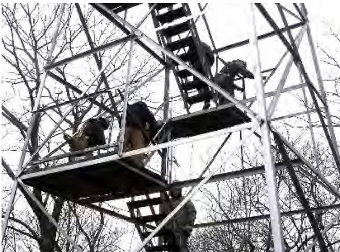
*Ironworkers installing new hand and mid-rails.*
