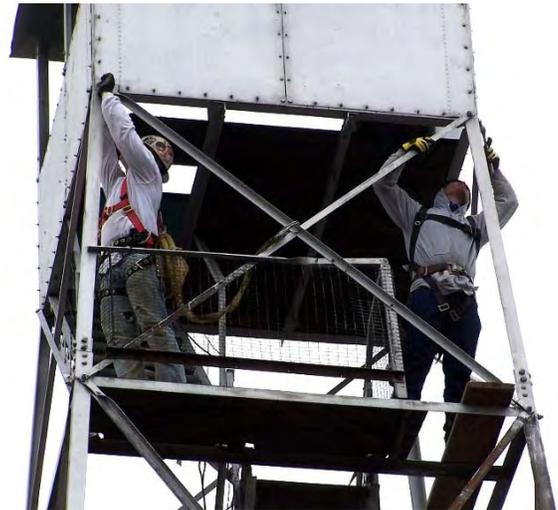
*Replacing "X" brace bolts and nuts*
