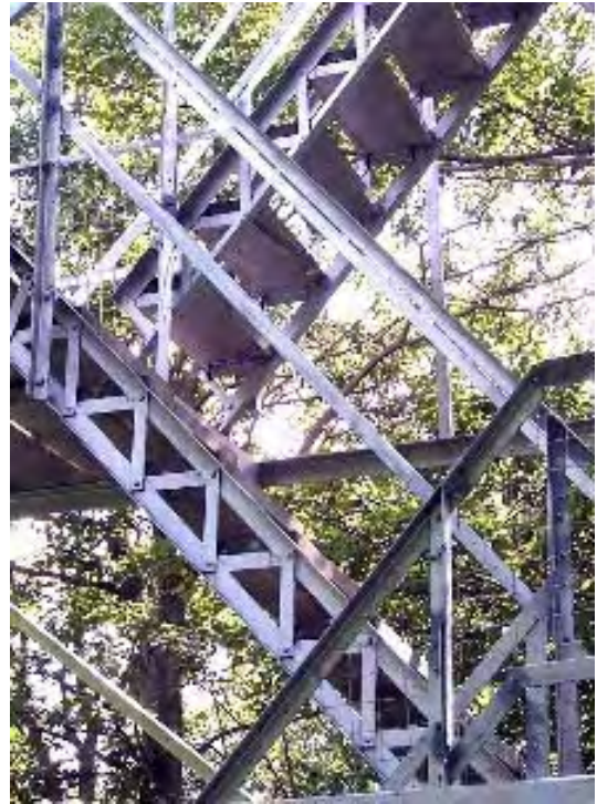
A new mid-rail on the second stair riser.
