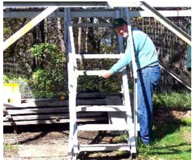
Chapter member Mark Haughwout securing stair treads.
