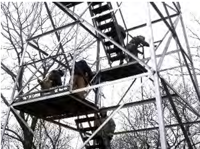
Ironworkers installing new hand and mid-rails.
