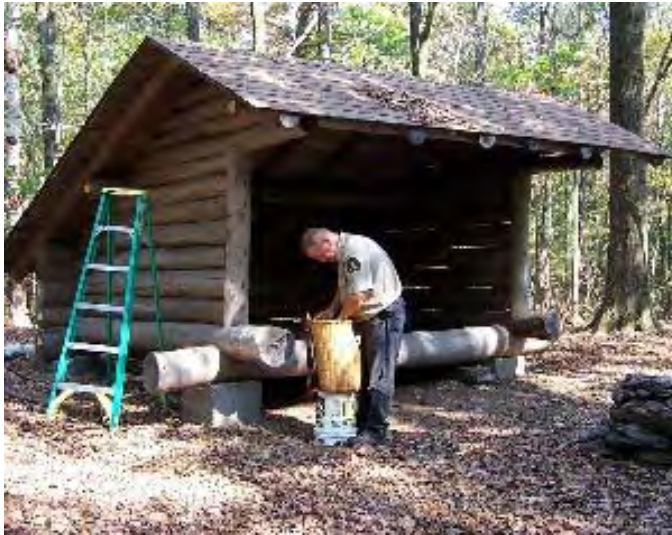
FFLA state director Bill Starr preparing to apply the linseed oil stain to the lean-to.
