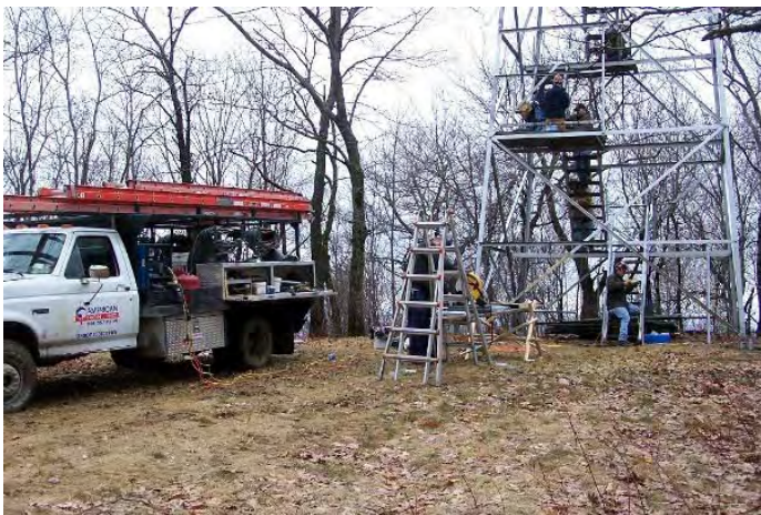
On site part fabrication
