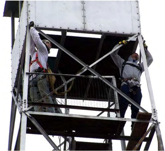
Replacing "X" brace bolts and nuts
