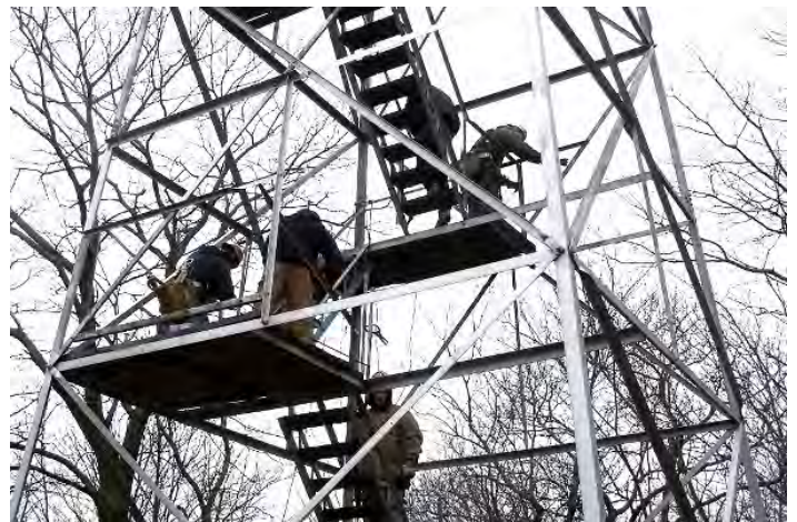
Raising the hand rail elevation to 42"
