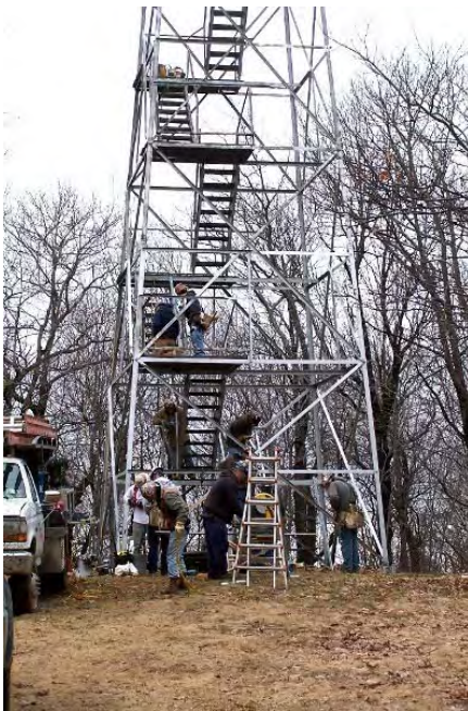
Ironworkers preparing to start work.
